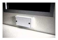
1) Remove the lid seals acting on the two screws by with Allen key which is provided. Do the same action inside the booth.
