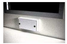
1) Remove the seal acting on the two Allen screws with the provided wrench. The same operation must also be performed within the booth
